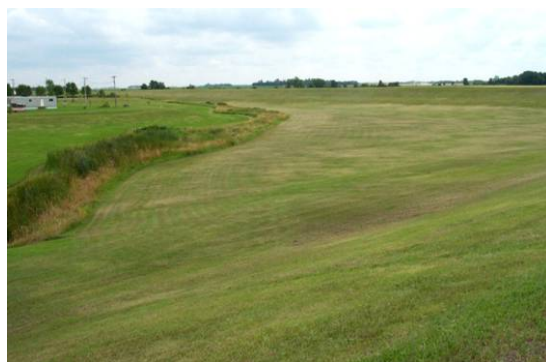
Figure 2.57 ACCEPTABLE interior ponding area and drainage ditch. (MN)
