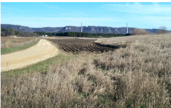
Figure 2.6 UNACCEPTABLE levee encroachments. This landowner tilled near one third of the way up the landward levee slope. (MN)
