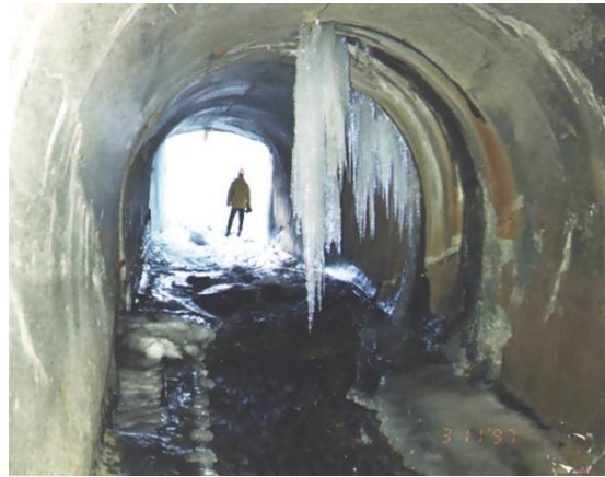
Figure 2.58 Concrete drainage tunnel. (AK)
